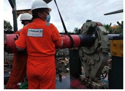
Set Up Casing and Tools Before Make up Torque process
