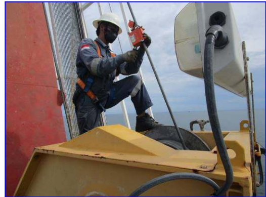
Perform WRT of Auxiliary Hoist
